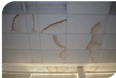
Leaky and damaged roofs must be repaired or replaced.
