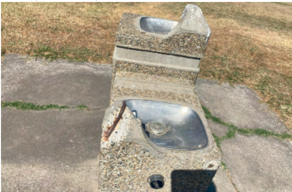
Drinking fountains are broken/damaged
