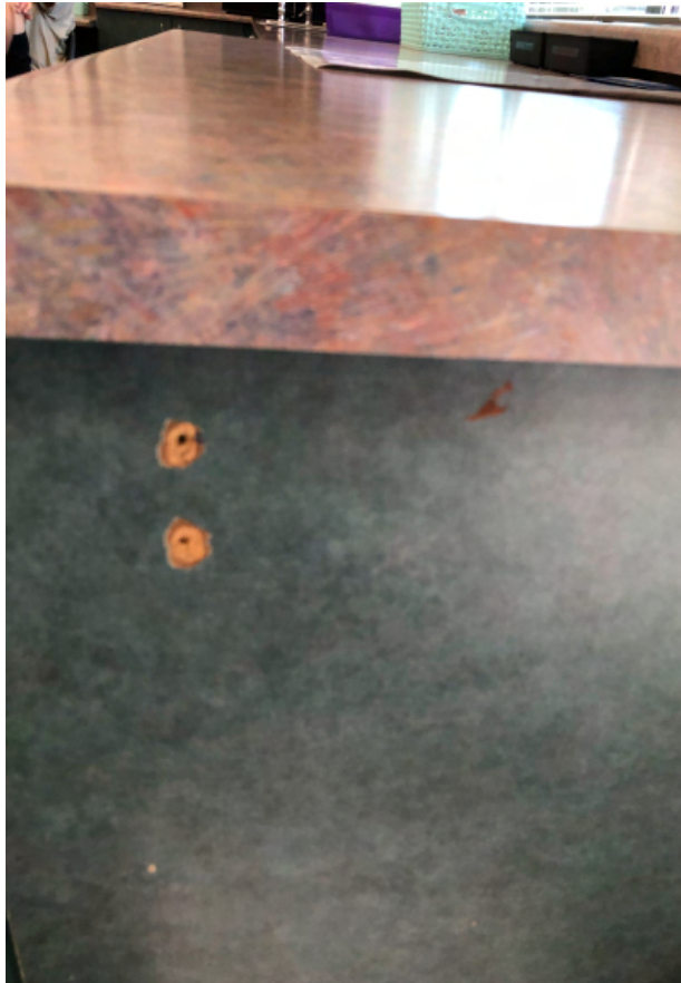
Damage to casework in classrooms
