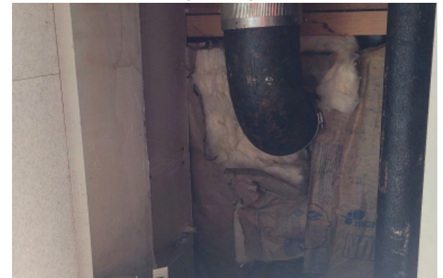
Exposed wall internals
